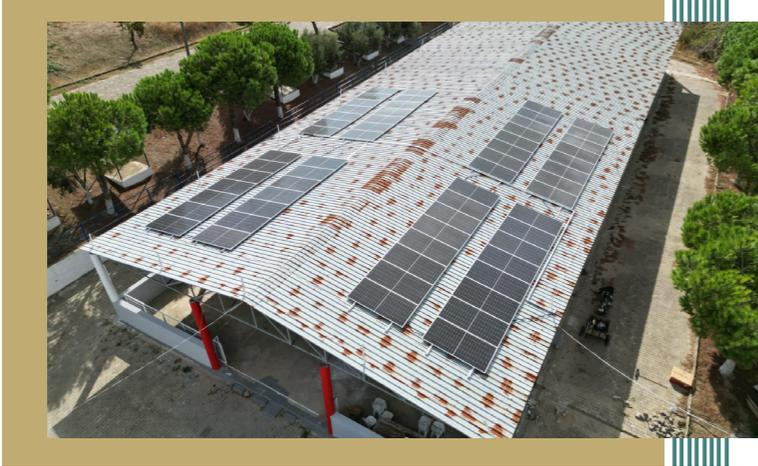
Over 120 solar panels, which produces 50kW of power, were installed on the roof of Kavakköy Municipality Covered Market Place. It was aimed to produce approximately 94,000 kWh of energy annually and decrease the energy expenses of the Municipality. In addition, the facility is connected to the national grid to transfer excess electricity.
