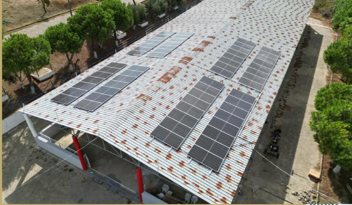
Over 120 solar panels, which produces 50kW of power, were installed on the roof of Kavakköy Municipality Covered Market Place. It was aimed to produce approximately 94,000 kWh of energy annually and decrease the energy expenses of the Municipality. In addition, the facility is connected to the national grid to transfer excess electricity.
