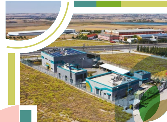
Main Control Center (MCC) Ankara
