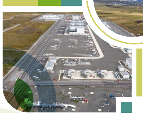
Compressor Station (CS-1) Ardahan
