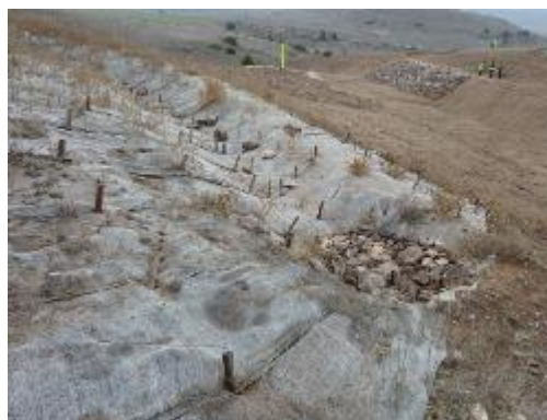
Figure 13 Rock lined slope breaker outlet at KP 1369
